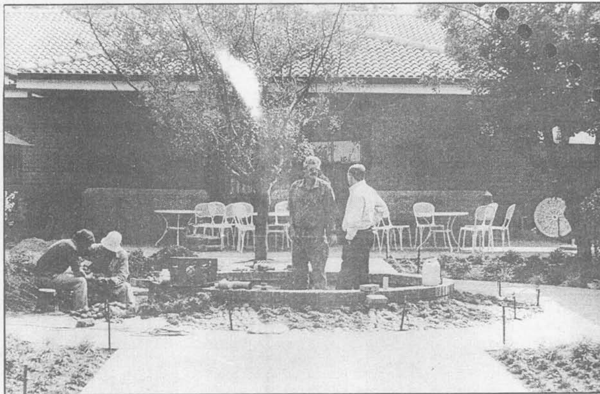
FABI's fabulous fish pond ..... during renovations
